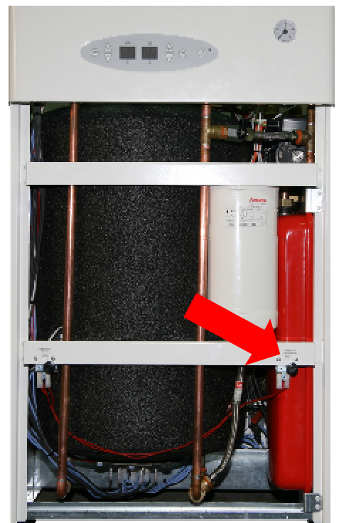
Location of the thermal limiter HEATING in a CVXP boiler.
