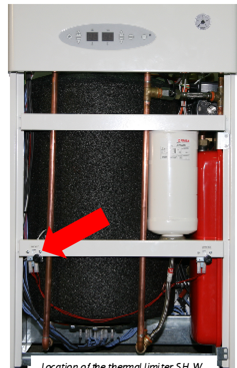
Location of the thermal limiter S.H.W. in a CMXP boiler.
